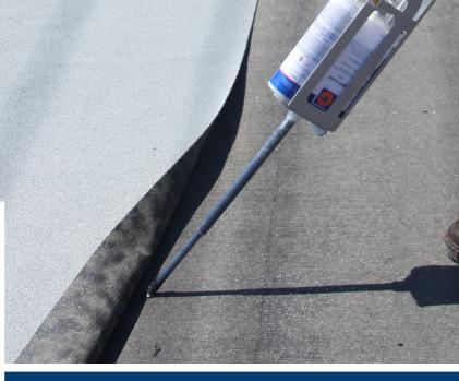
Night-Lock foam sealant provides a clean, secure seal for overnight watertight protection, making it the ideal night tie-in solution for active projects. The foam sealant is highly elastomeric, solvent free, quick setting and specially formulated to save time while keeping the job site protected. Night-Lock replaces asphalt mastics and bitumens or less reliable porous surface foams, significantly reducing the need for additional labor time and specialty materials.
