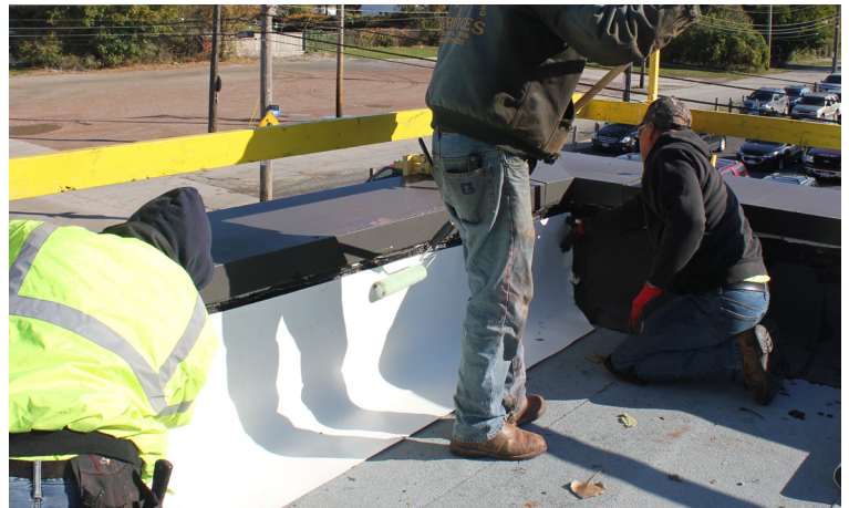
Membrane Installation
