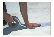
**Step 2** Apply pressure at the center of the tape and work toward the outside edge using a steel roller or hands. Press firmly to activate the bonding process and verify that all edges are tightly adhered with no gaps.
