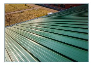
The high-performance clip and seam design on the R-Mer Shield system allows for unlimited thermal expansion and contraction to alleviate the effects of oil-canning and prevent seam buckling, resulting in a longer service life.
