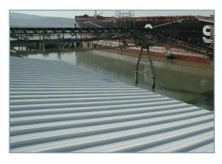
Separation of the sealant from the clip protects the system from the elements and prevents common concerns associated with thermal expansion and contraction, providing extraordinary watertight protection.
