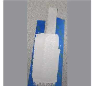
Apply coating, embed polyester fabric and saturate surface.
